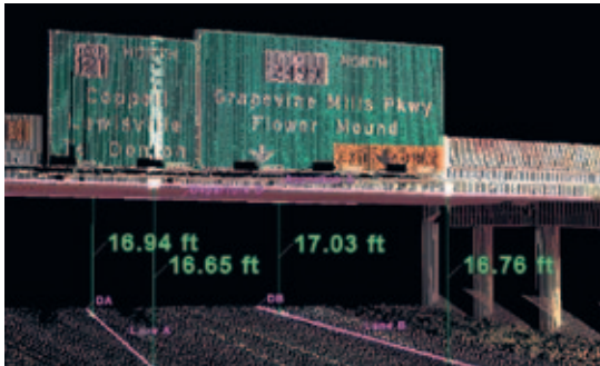
One of the many powerful measurement and annotation tools is an automated tool for analyzing and documenting clearances at overcrossings.
